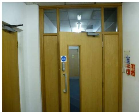
Views of the double fire doors on the corridor adjacent to the dance studio on the lower ground floor, without smoke seals fitted to the top and side edges.
