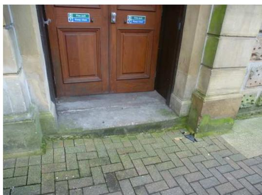
Views of the external steps to the side and front fire exits. These steps are a potential trip hazard.
