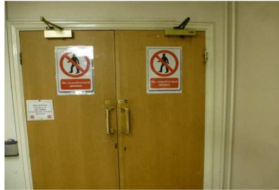
Views of the fire doors on the ground floor without smoke seals fitted to the top and side edges.
