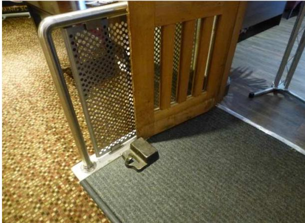
View of the fire door to the front room on the ground floor which is wedged open.
