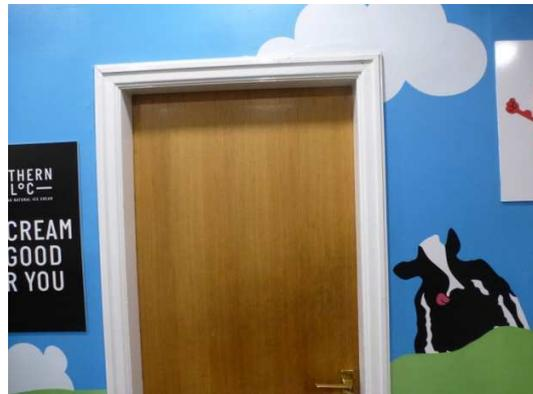
Views of the fire doors to the kitchen on the first floor, which do not have smoke seals fitted.
