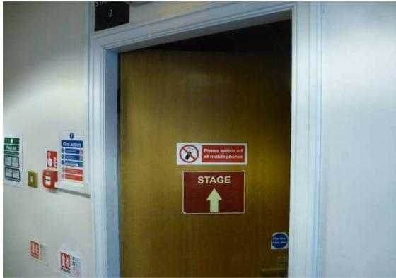
Views of the fire doors to the loft, control room and the stage door stairs on the second floor, which do not have smoke seals fitted.
